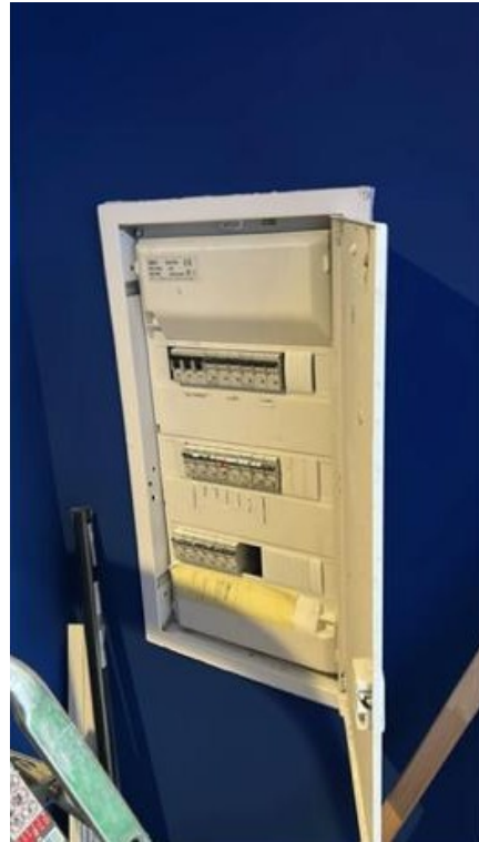
After: the new panel on the blue wall
